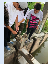
Setting the indicator into the channel
